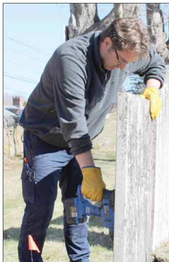
Once straightened, Kai Nalenz uses a modified hammer drill to tamp soil around the stone.
