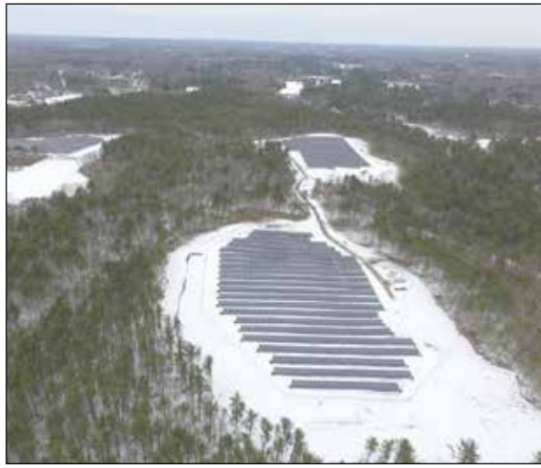
Submitted Photo by Lucas Faria This solar farm was built in Mendon. The property was previously undeveloped forested land and partially used for farming. The total system size is about 4.1 MW DC.
