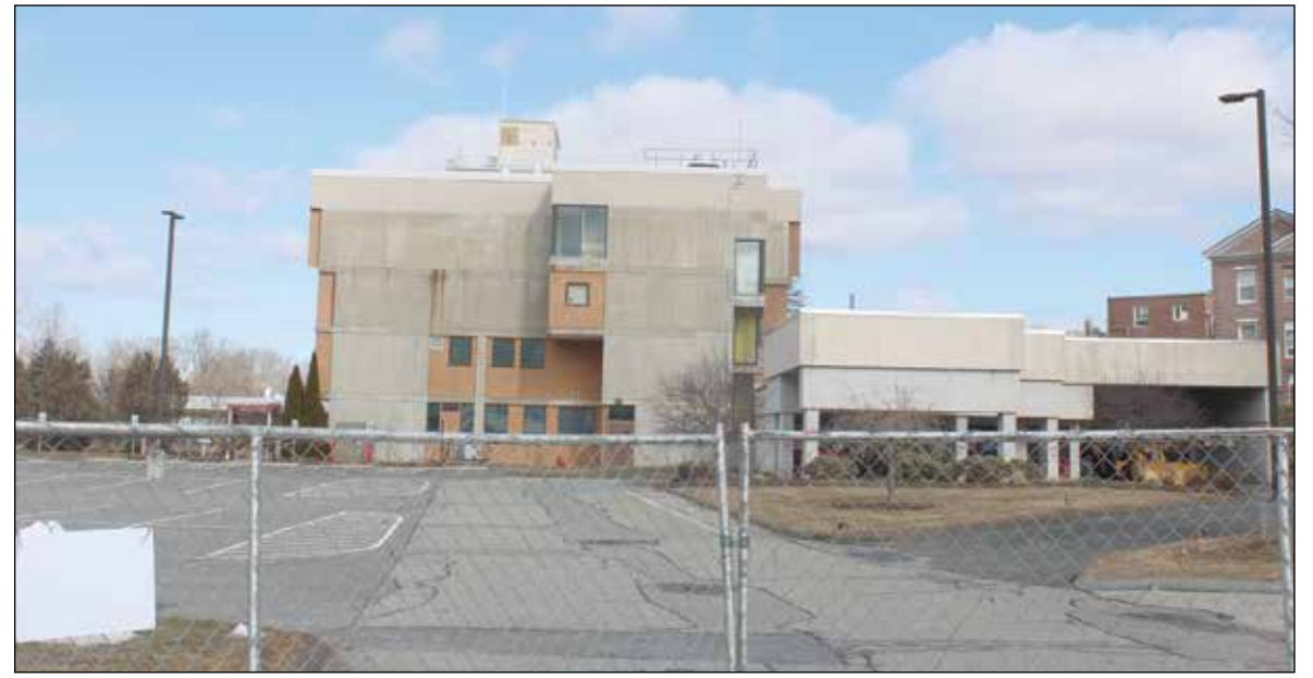
Turley Photo by Ryan Drago Baystate Mary Lane Hospital has been closed since the fall of 2023 and the site is currently under a nine-month demolition delay. This view of the site is from its entrance off Marjorie Street.
