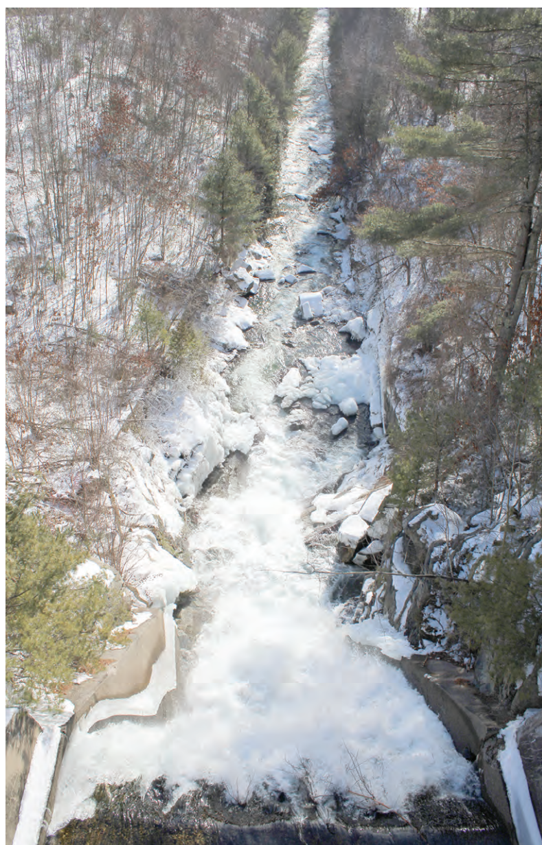
The lower spillway creates a waterfall, and only releases water when the Quabbin Reservoir is at or near capacity.
