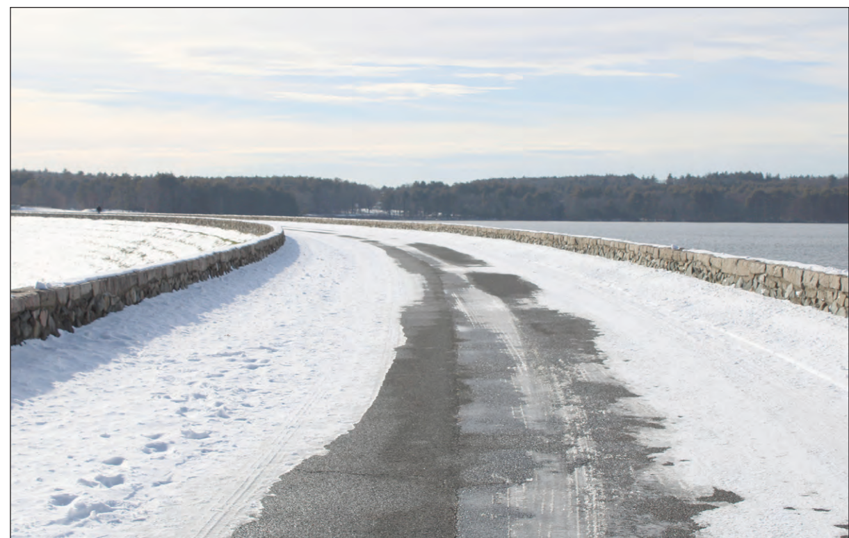
A roadway passes over the top of Winsor Dam. Although it is no longer open to public vehicles, walkers and bicyclists are welcome to explore the massive structure.
