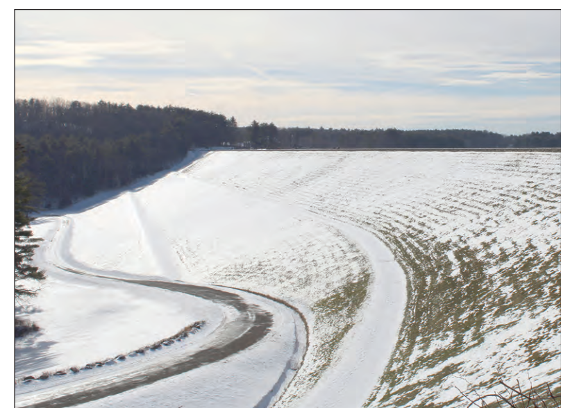
There are 40 caissons buried under this impoundment.
