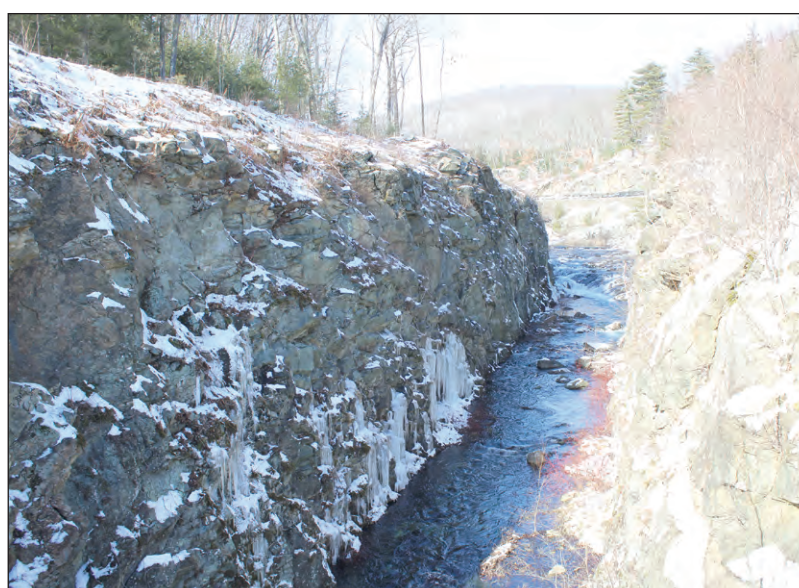
The spillway was formed by blasting rock.
