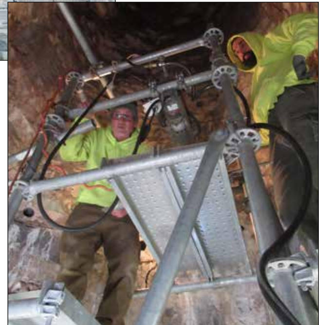
This photo shows the scaffolding at the Stone Church for Phase 4 Lantern Level interior stabilization.
