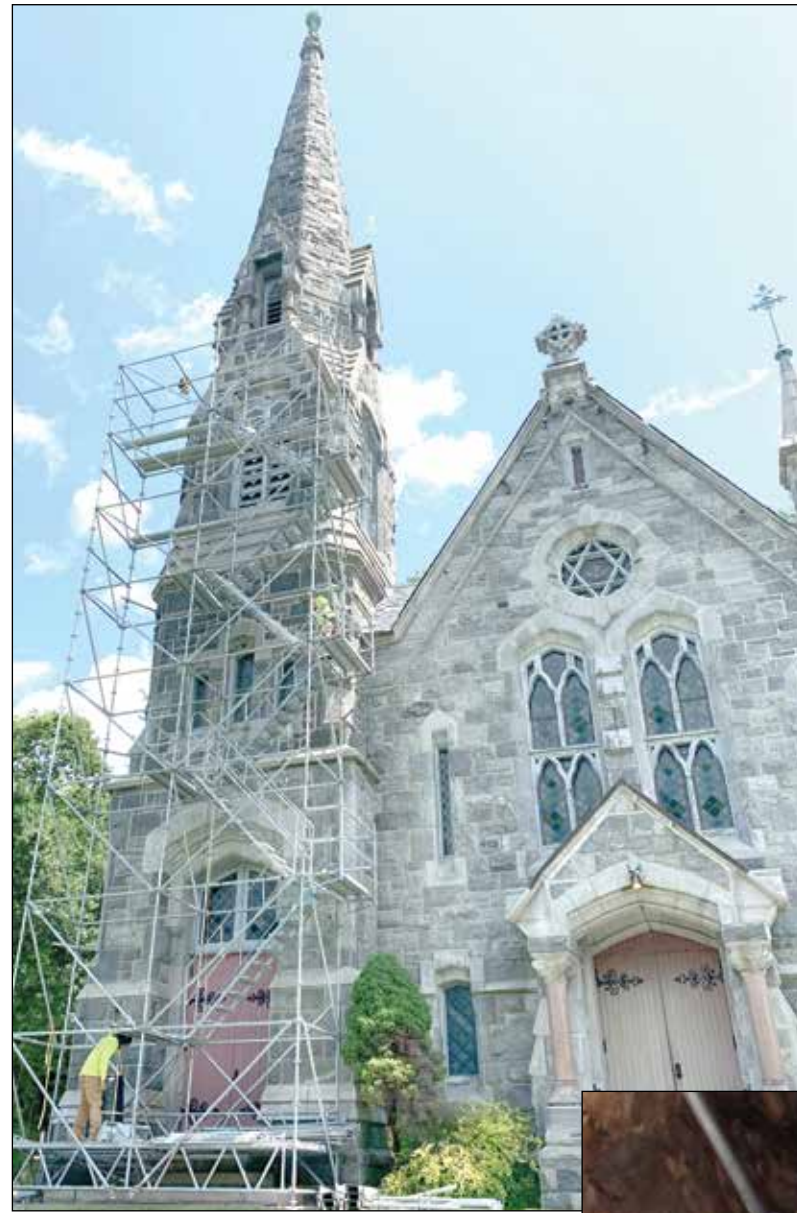
This photo shows the scaffolding at the Stone Church for Phase 4 Lantern Level interior stabilization.
